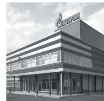
СК «ГАЗПРОМ ПРОМЕТЕЙ» Construction Company "Gazprom Prometheus"
